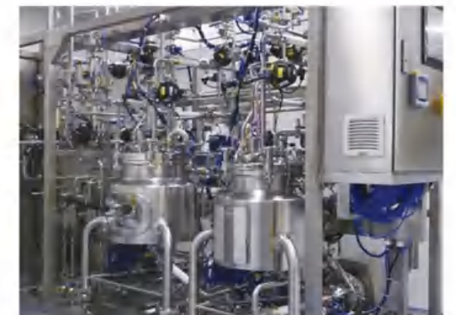
制药行业DE-CIP安装 DE-CIP installation in the pharmaceutical industry
